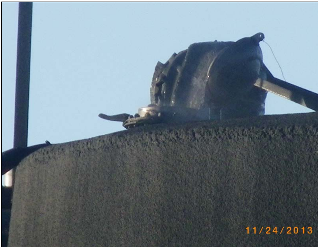
And another site showing the tanks with open hatches:
